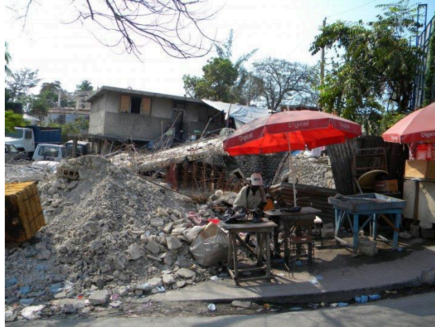
Houses and buildings were “pancaked” by the earthquake, Port au Prince, 2010
