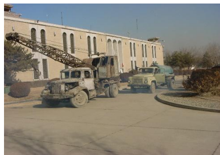
Vehicles and supplies arrive via Antonov; the one working toilet and shower; old Embassy equipment used to dig sewers, reinstate electricity and water, remove debris
